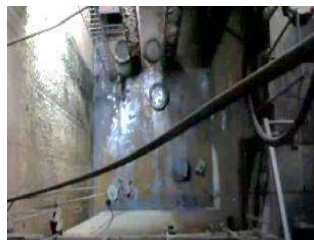
Technological vault metal constructions dismantling
