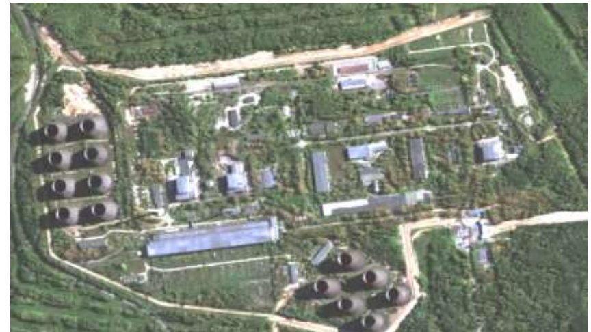
South site (area 2) - 3 industrial reactor plants
