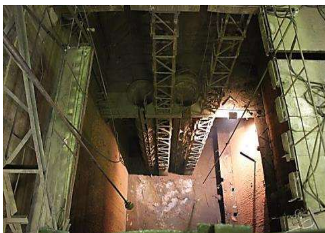
Technological vault metal constructions dismantling
