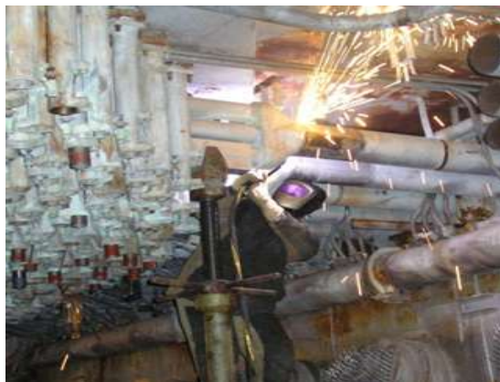
Utility systems pipelines dismantling
