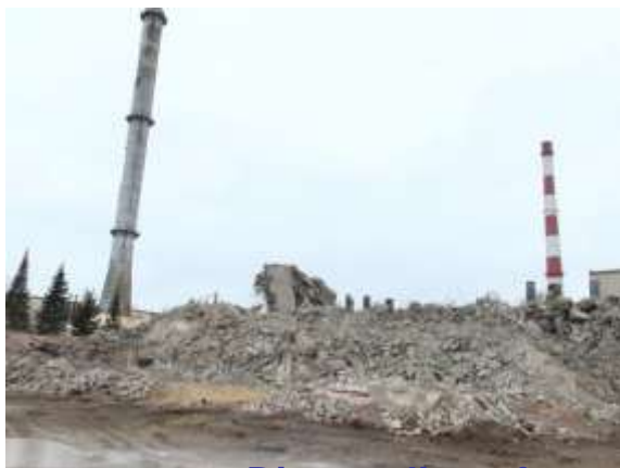
Dismantling of central hall engineering structures
