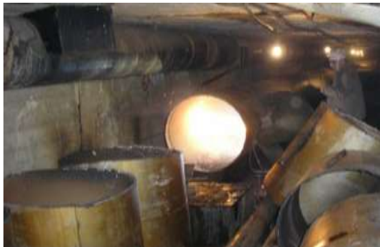
NPP first circuit pipelines dismantling
