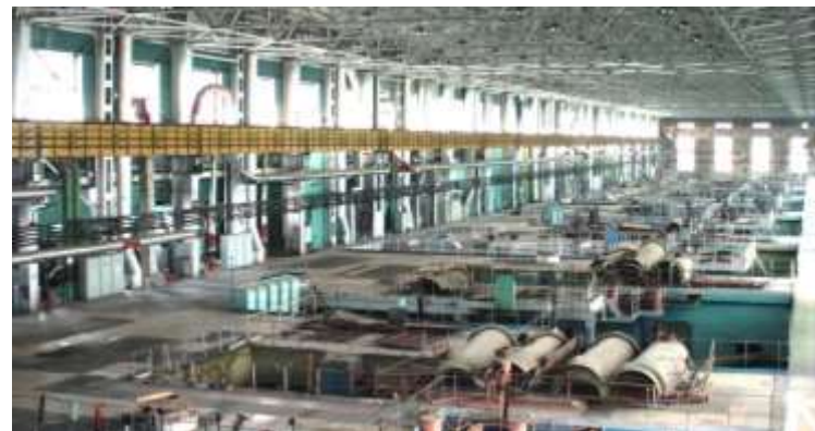
NPP heating equipment dismantling
