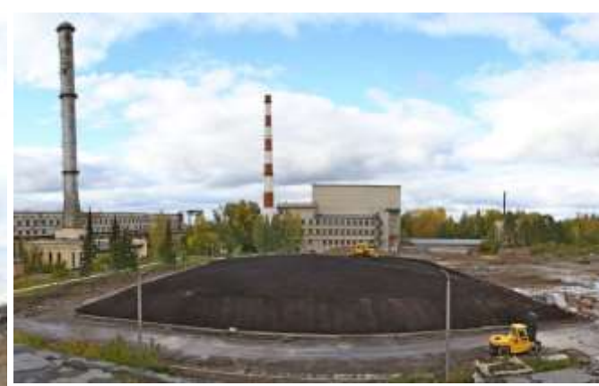
Construction of protective shield
