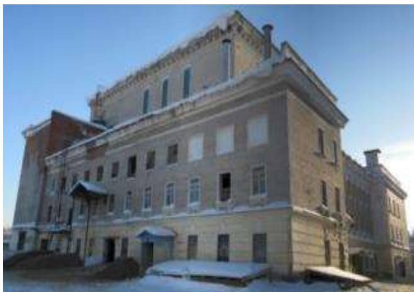
External appearance of EI-2 reactor in 2012 before D&D
