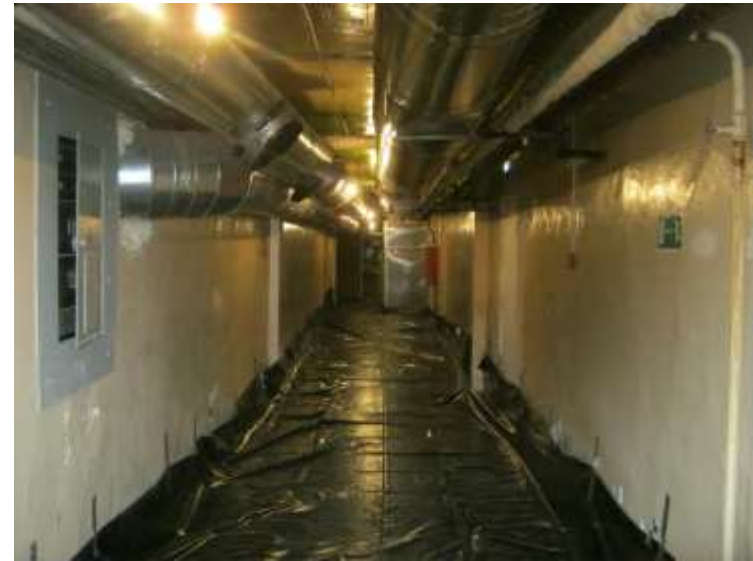
Decontamination of interior rooms and systems
