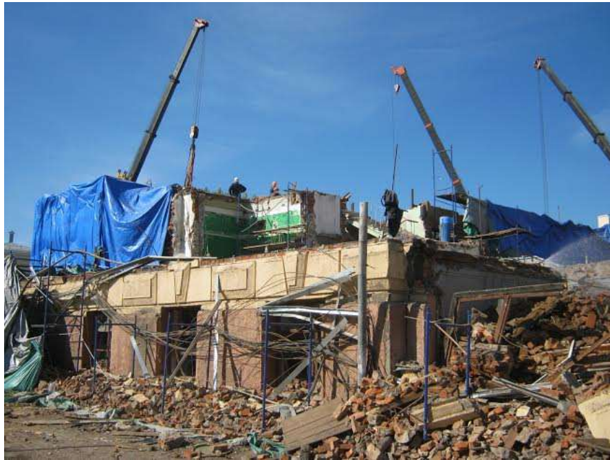
Dismantlement of building structures
