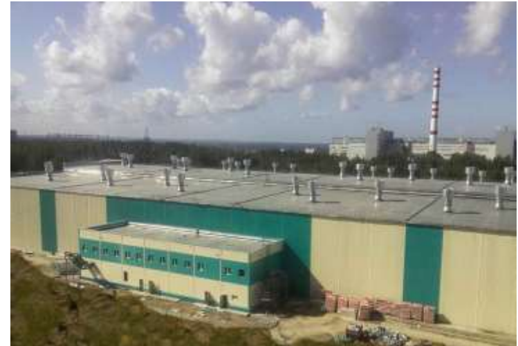
Module storage of solidified liquid RAW (building 667a)
