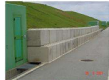
Consolidation of slope
