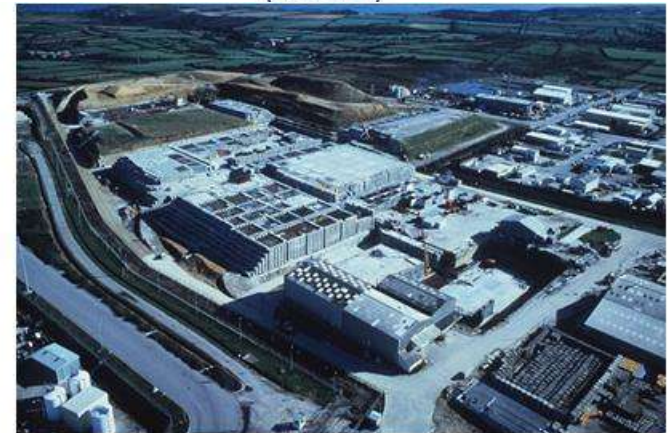
The site (1991) with disposal platforms
