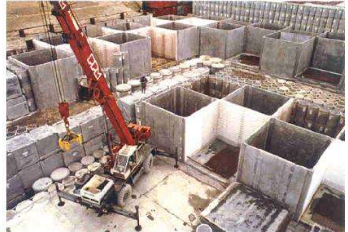
Disposal platform and cells to be grouted (1985)
