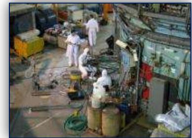
Reactor bioshield drilling and sampling
